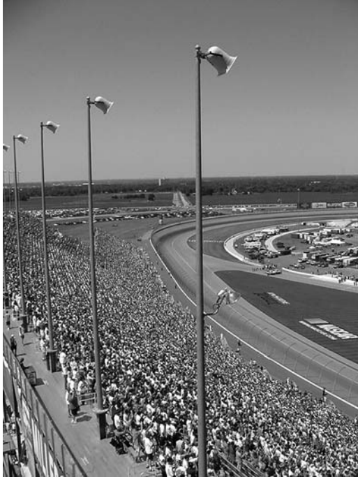
Figure 34-87. Outdoor-rated loudspeakers at a motor race track. Courtesy Community Professional.
