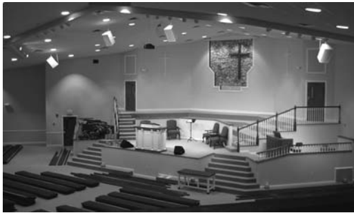
Figure 34-19. An exploded cluster loudspeaker system. Courtesy Community Professional.
