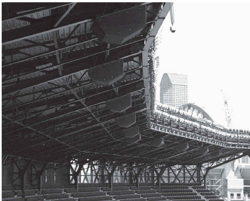
Figure 34-82. Distributed clusters in a stadium. Courtesy Seattle Mariners.
